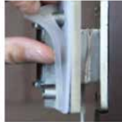
Rubber against glass, plastic against hinge plate.
